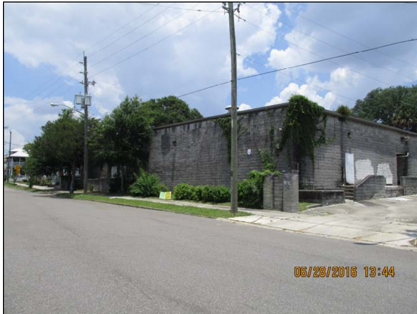
Non-contributing warehouse on Pearl Street to be demolished.
