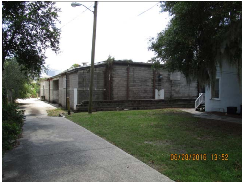
Western-most alley connecting the project to W 4 th Street.
