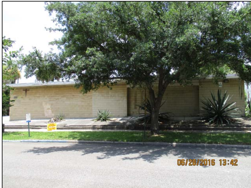
Non-contributing dentist's office to be demolished.
