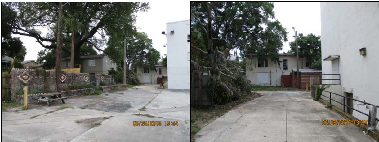
Interior parking area, behind Building D and Building E.
